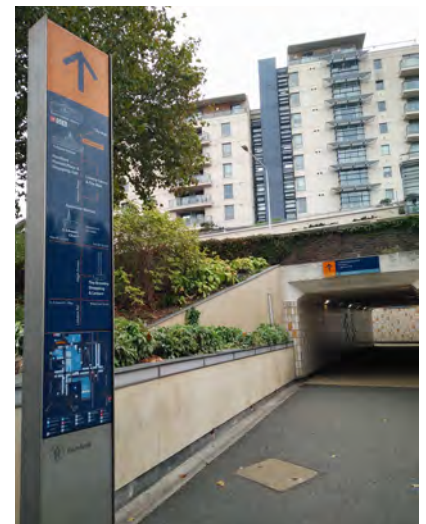
O4 - Romford Roundabout underpass
